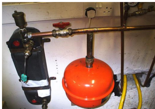
Figure 16: The connections of the heat exchanger and expansion valve.
