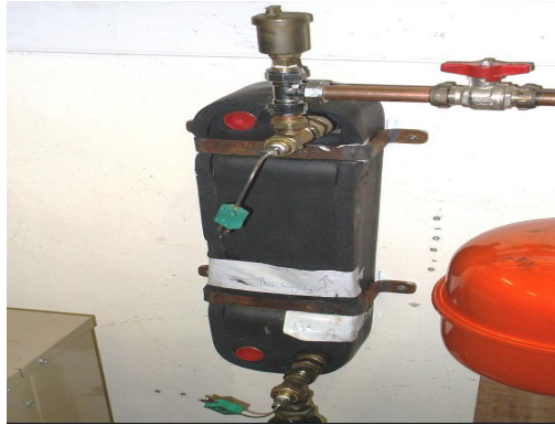
Figure 14: The heat exchanger.
