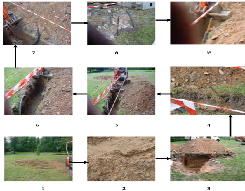
Figure 3. Drilling (1-2) digging of the pit (3), connection of the manifolds (4), grouting, preparation of the coils (5-6) and the source loop, which consists of two earth loops: one for vapour and one for liquid (7-9).
