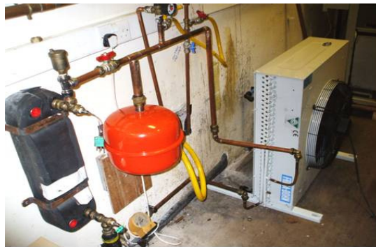
Figure 15: The connections of the heat exchanger, water pump, heat rejection fan and expansion valve.
